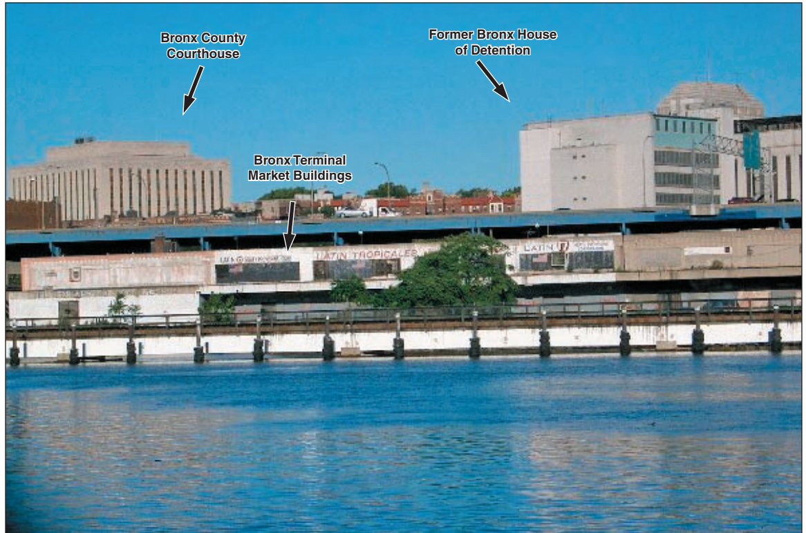
View northeast from the Esplanade Gardens (Lenox Avenue and West 147th Street) in Harlem. The Bronx Terminal Market portion of the project area is in the foreground
