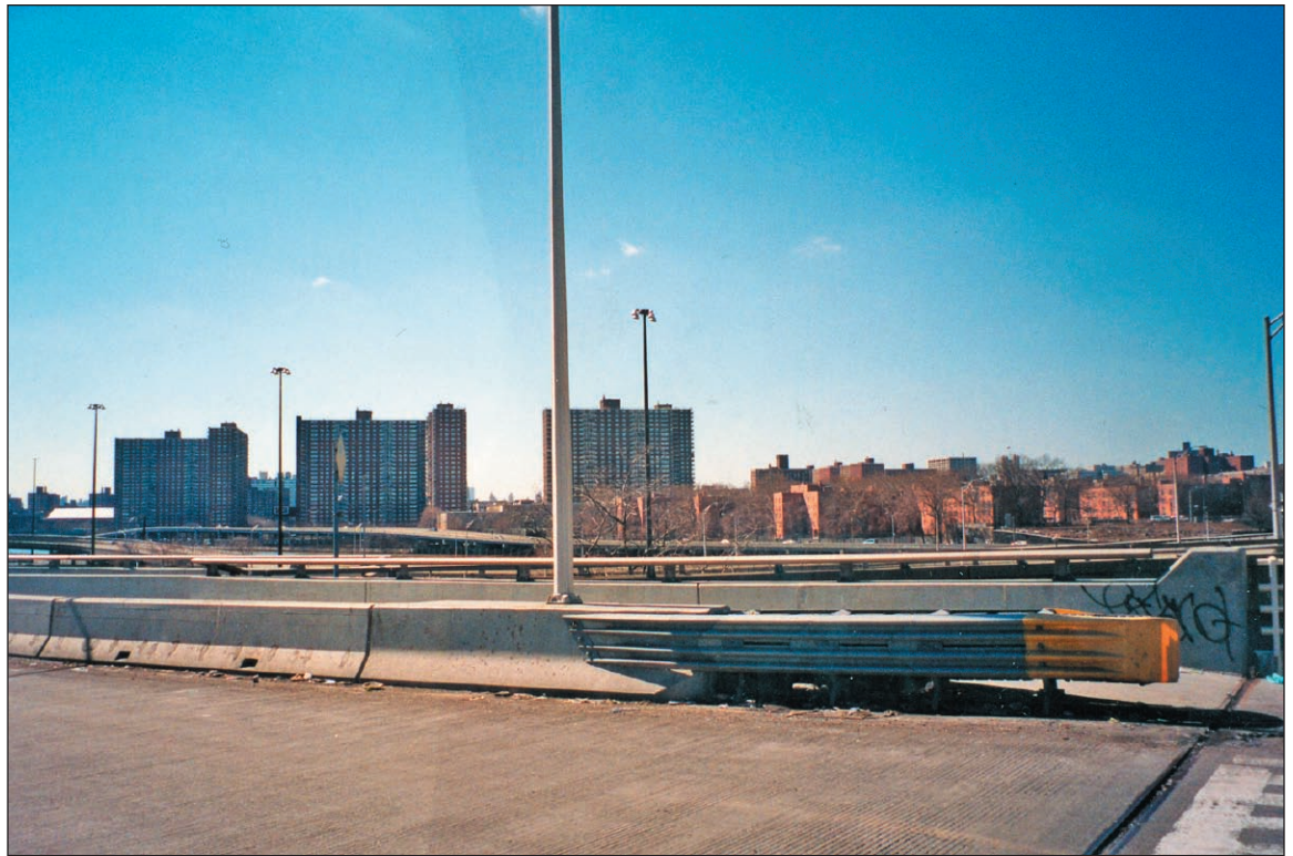
Macomb's Dam Bridge Approach, view west 42
