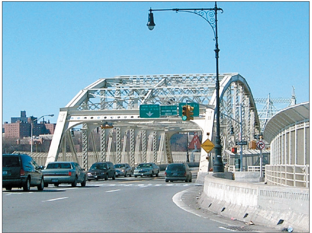
Macombs Dam Bridge, Metro-North right-of-way span 10
