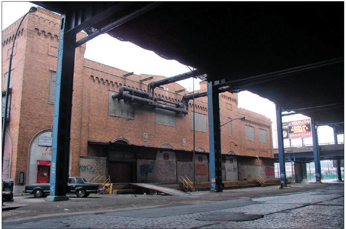
Bronx Terminal Market, Building J 8
