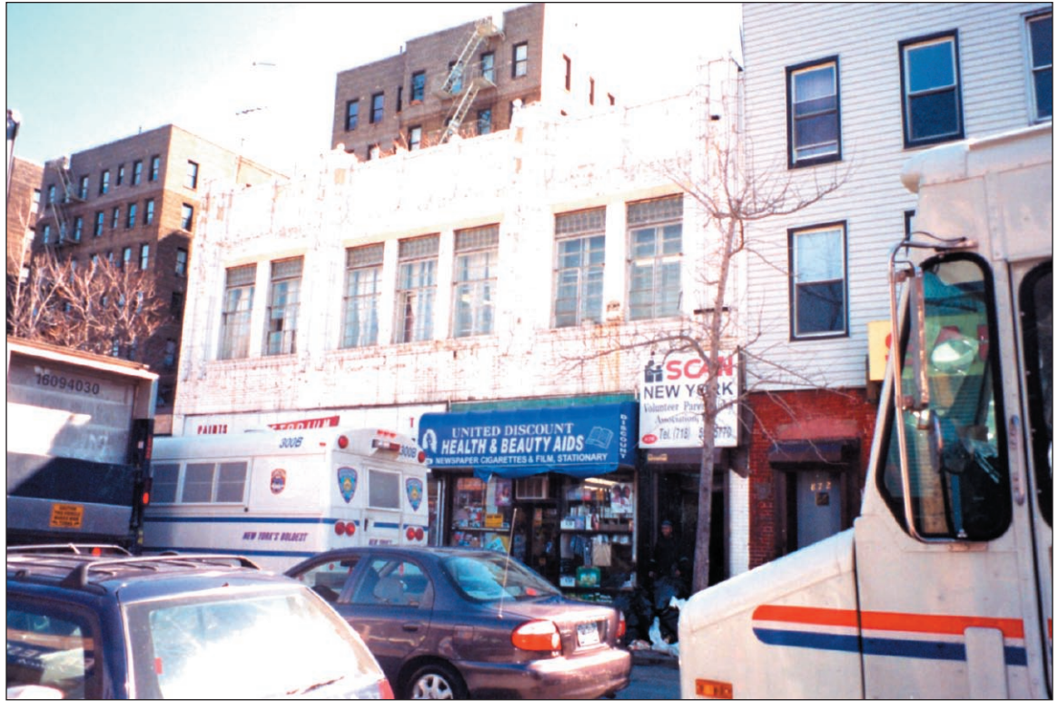
876-878 Gerard Avenue/893-895 Walton Avenue, west facade 31
