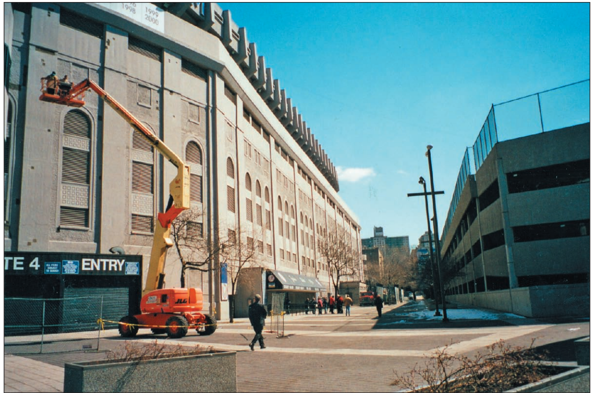
Yankee Stadium, view east on East 157th Street 4
