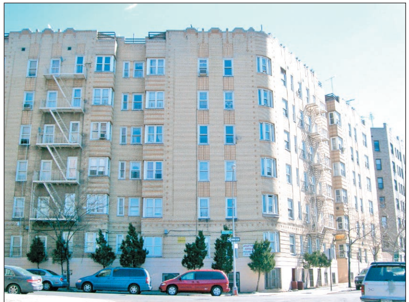
690 Gerard Avenue at East 153rd Street 30
