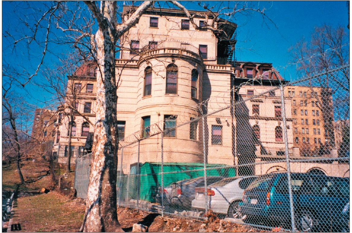
View west on Jerome Avenue from Anderson Avenue 41
