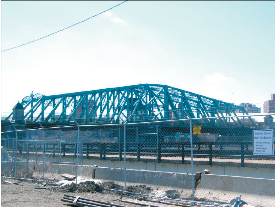
145th Street Bridge 17
