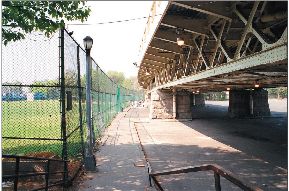
Macomb's Dam Bridge Approach 12
