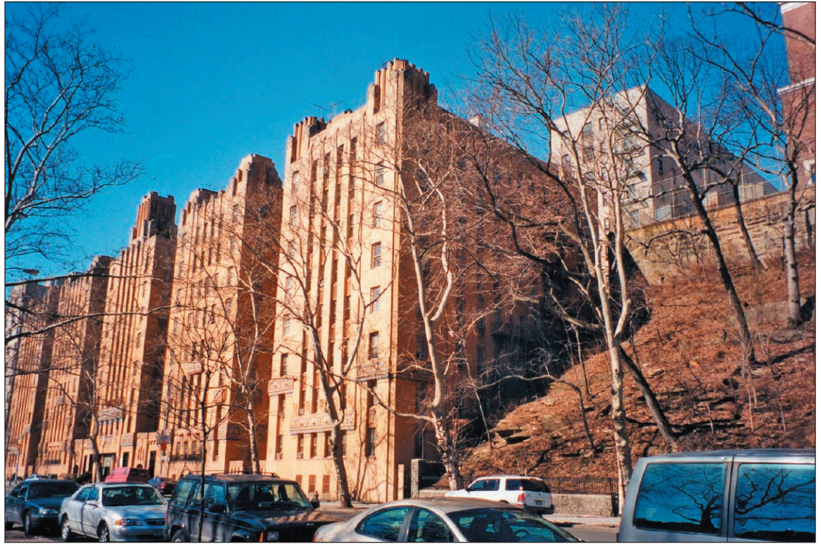
View southwest on Jerome Avenue from East 165th Street 40
