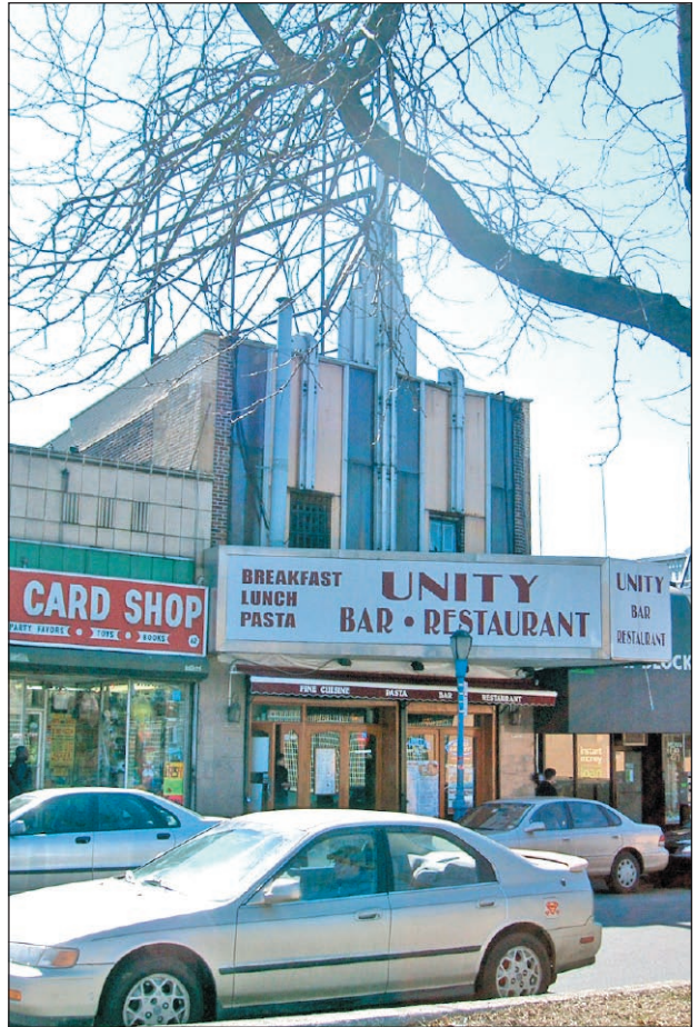
58 East 161st Street, north facade 25
