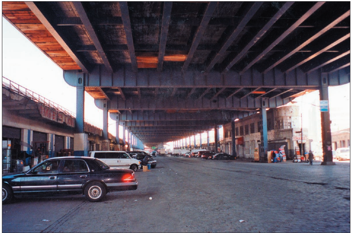
View north on Exterior Street from East 150th Street 30
