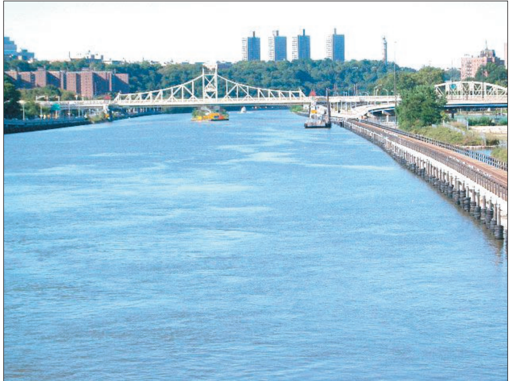
Macombs Dam Bridge, Harlem River span 9
