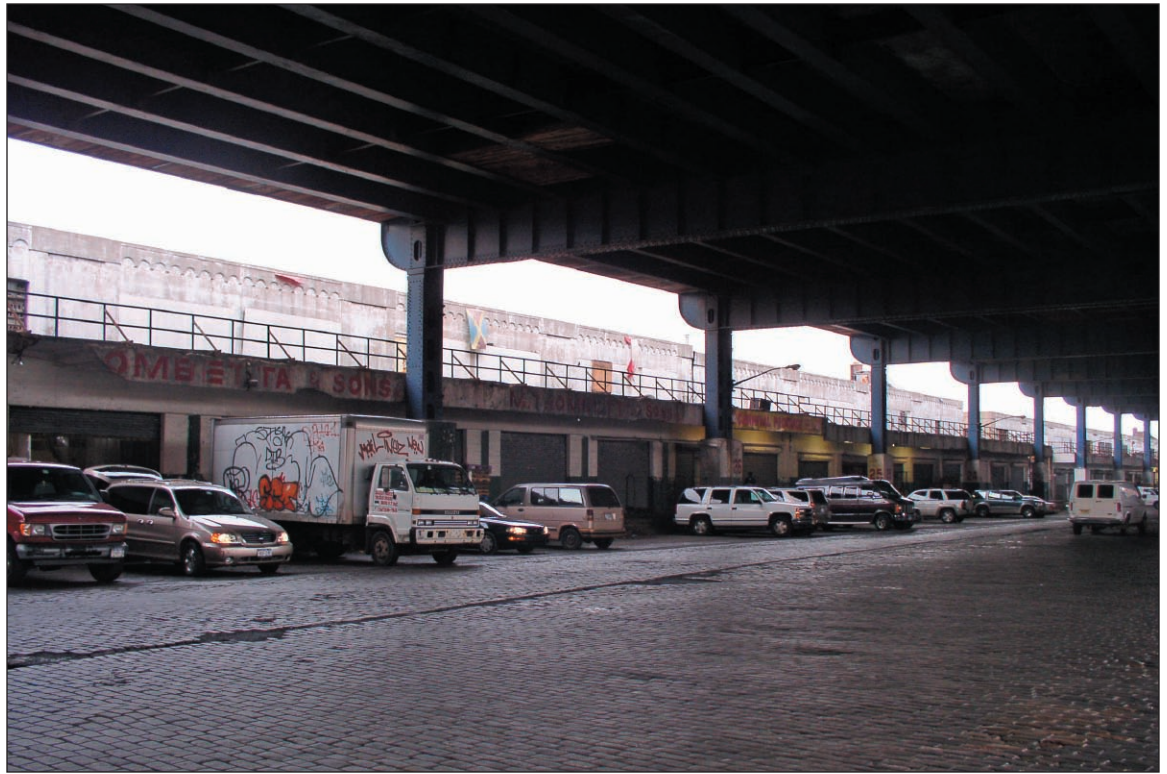
View northwest of Bronx Terminal Market Buildings F/G/H 15
