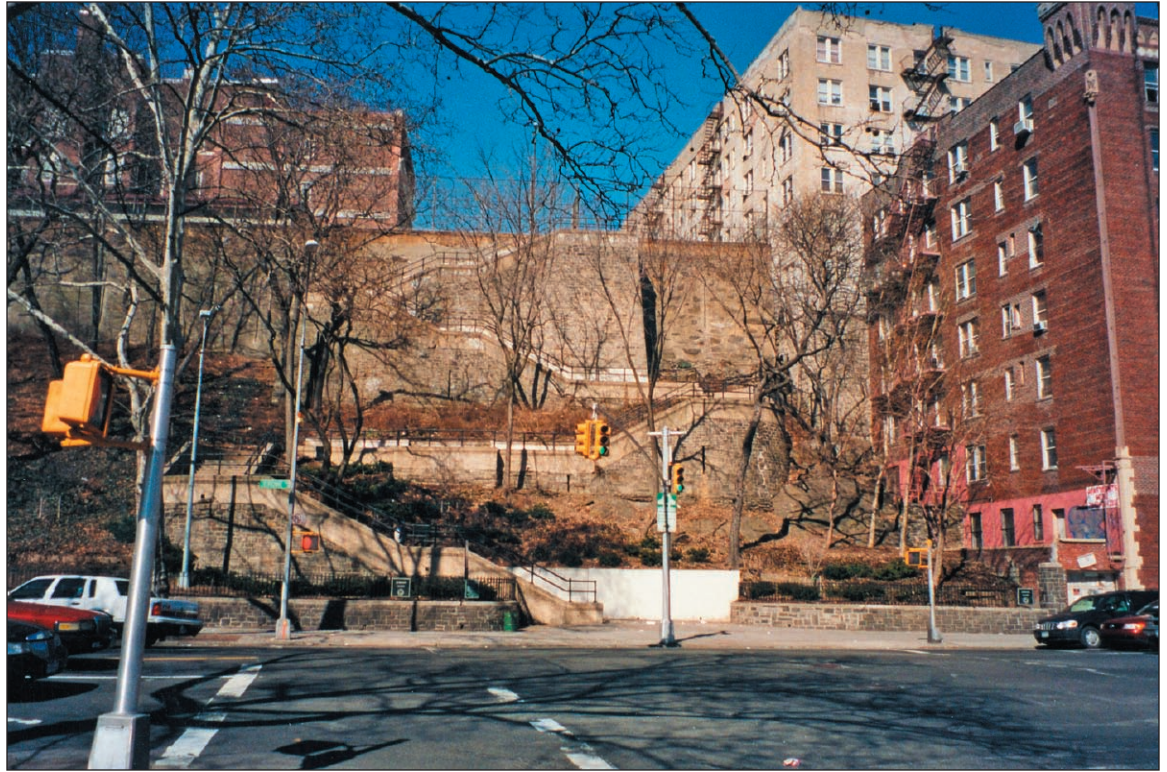
View west of Jerome Slope from East 165th Street 23
