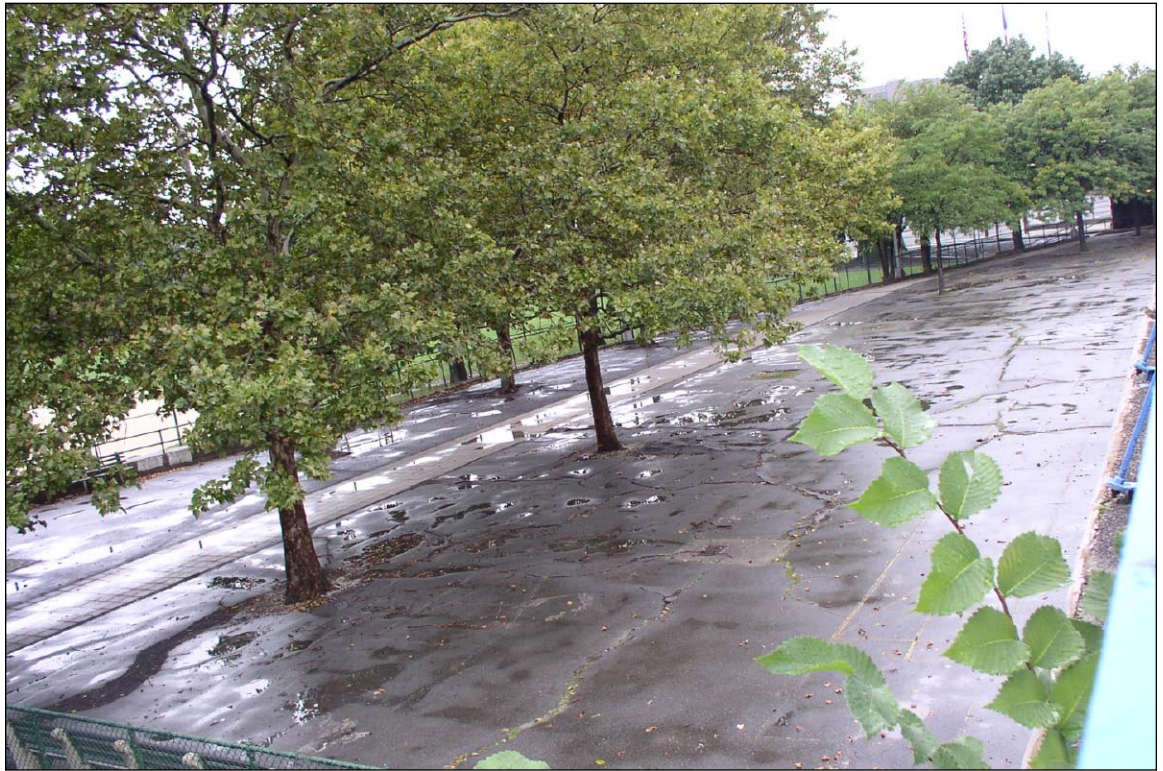
Plaza area at southern portion of Maccomb's Dam Park 4
