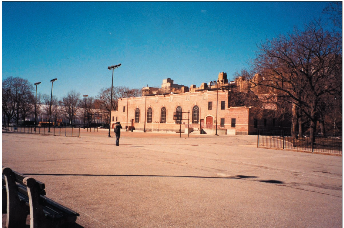
View southwest of the west side of John Mullaly Park 34
