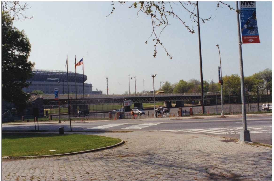
View southeast from 161st Street and Jerome Avenue. The Macombs Dam Bridge crosses the project area as an elevated stone and steel structure
