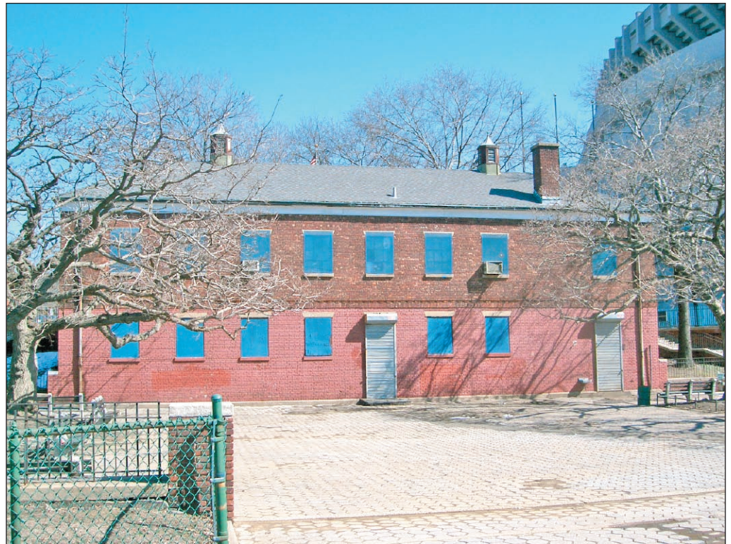
Maccomb's Dam Park District Office, southeast facade 5
