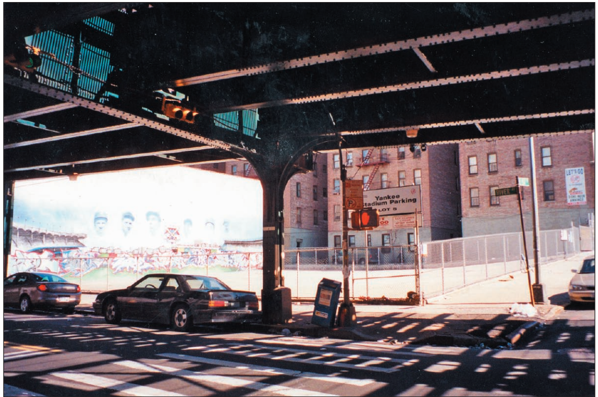
Parking lot at the northeast corner of River Avenue and East 157th Street 18
