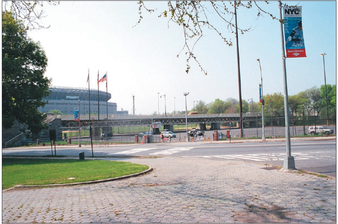
Macomb's Dam Bridge Approach 11
