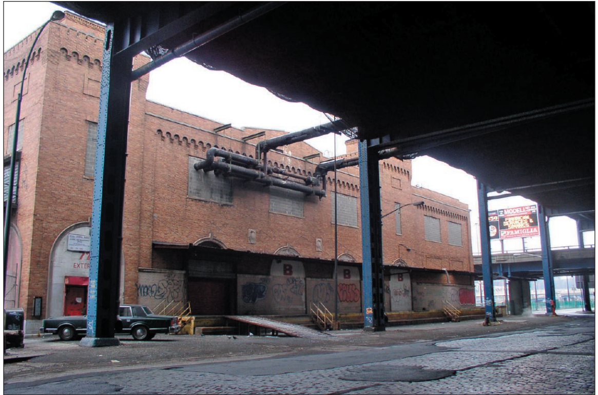
View northwest of Bronx Terminal Market Building J 14
