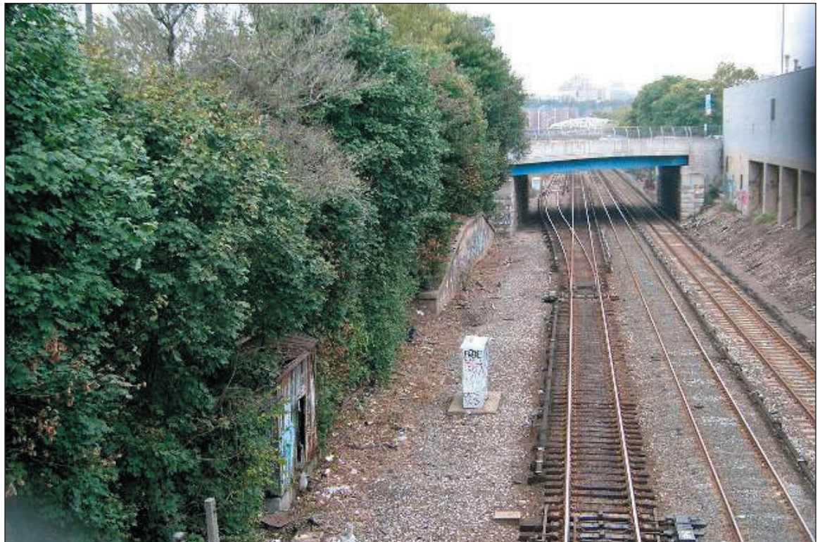
Metro North Railroad right-of-way, view west from Gerard Avenue between East 151st and East 153rd Streets 32
