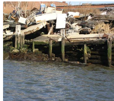
FIGURE 2-10: TIMBER CRIB WALL, BUSHWICK INLET
