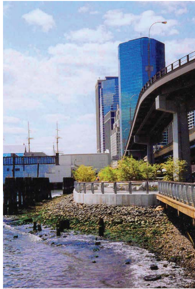
FIGURE 6-32: RIPRAP AND CURVED BULKHEAD WALL
