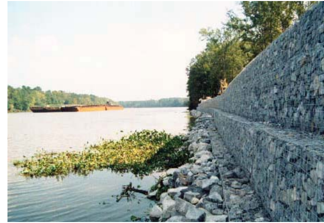
FIGURE 6-33: RIPRAP AND GABION WALLS, PHOTO COURTESY OF THE INTERNATIONAL EROSION CONTROL ASSOCIATION
