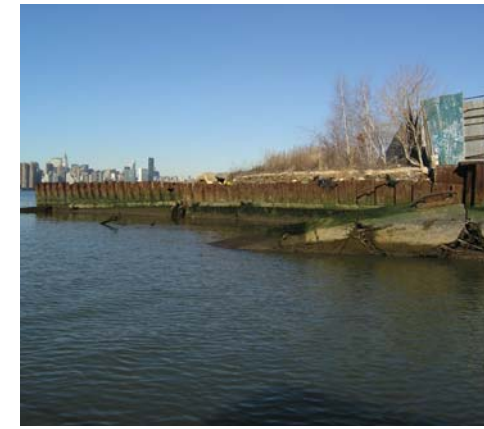
FIGURE 2-8: STEEL SHEET PILE BULKHEAD AT N. 4TH STREET
