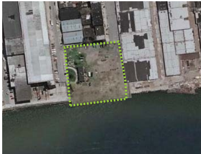
FIGURE 5-10: TRANSMITTER PARK, EXISTING SITE
