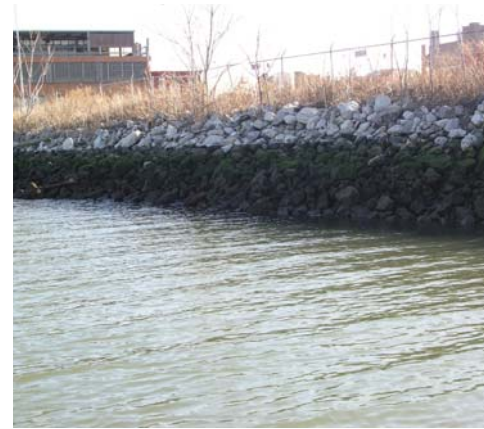
FIGURE 2-6: STONE RIPRAP SLOPE, KENT STREET
