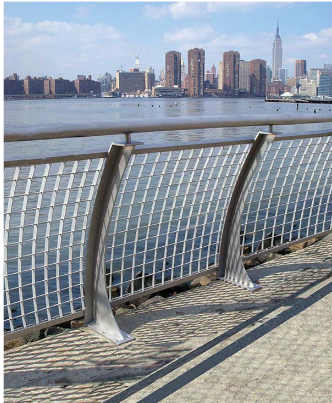
FIGURE 6-12: WATERFRONT WXYRIVER RAILING
