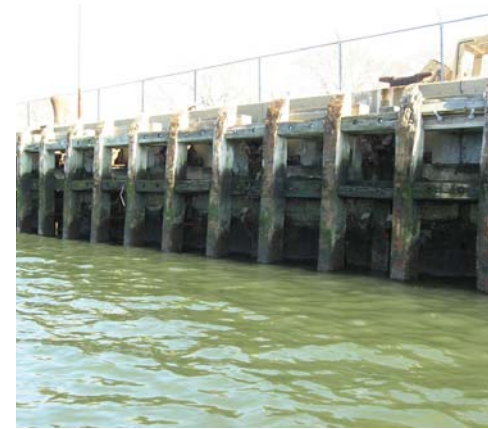
FIGURE 2-7: TIMBER BULKHEAD WALL, MANHATTAN AVE.
