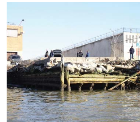
FIGURE 2-11: LOW-LEVEL PLATFORM, HURON STREET
