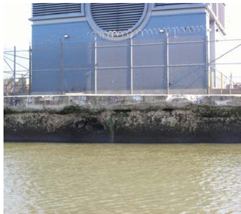
FIGURE 2-9: CONCRETE SEAWALL, N. 7TH STREET
