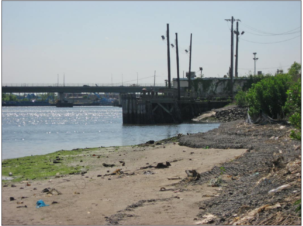
Intertidal unvegetated shoreline along the north shore of Main Creek at Creek Landing. Rip-rap and gabions being used to stabilize the shoreline 15
