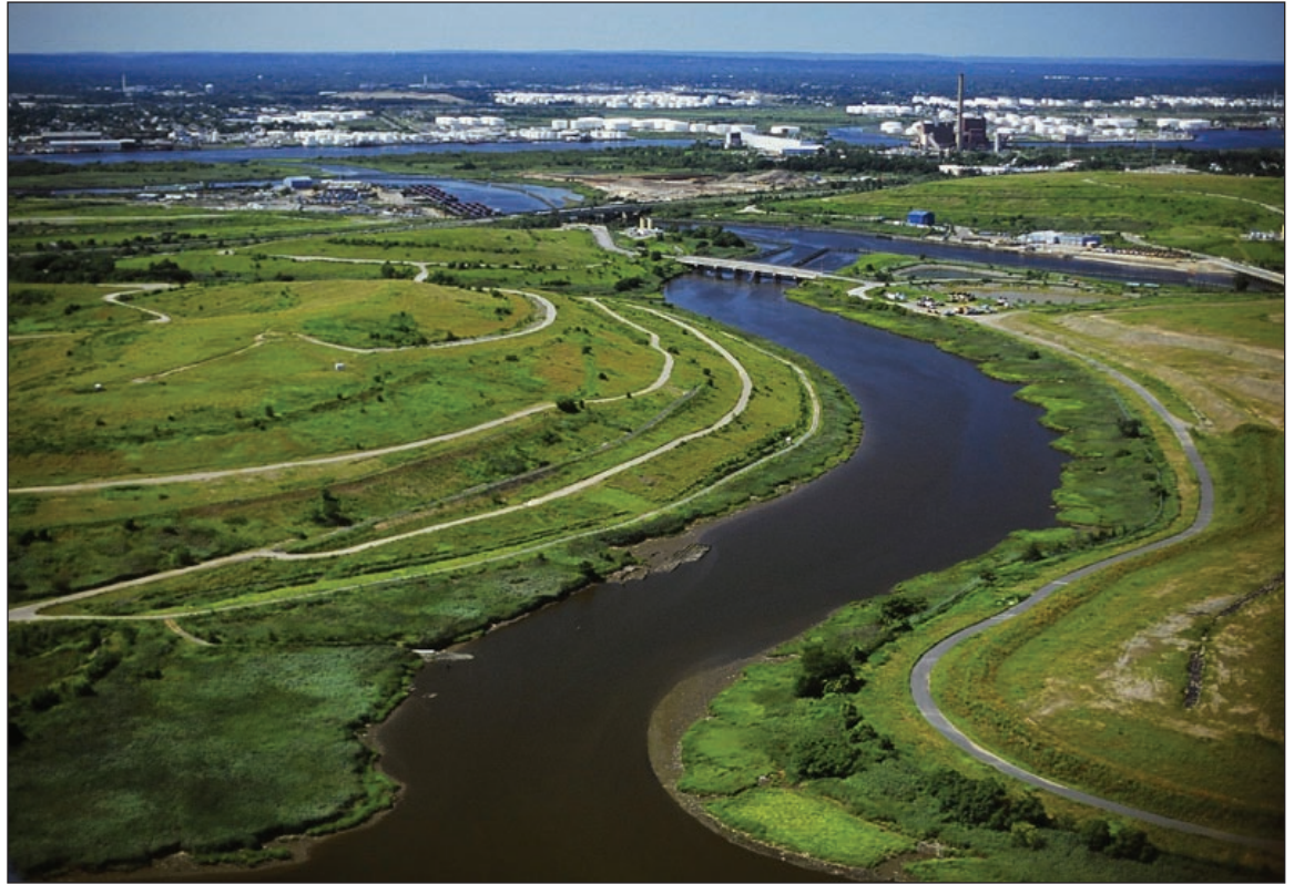
DSNY access roads traverse the site in response to mound shape 1
