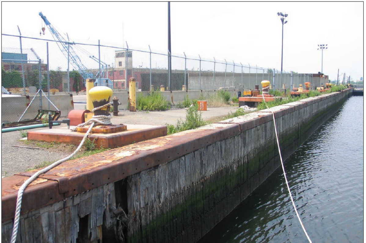
Bulkheads at Fresh Kills 13
