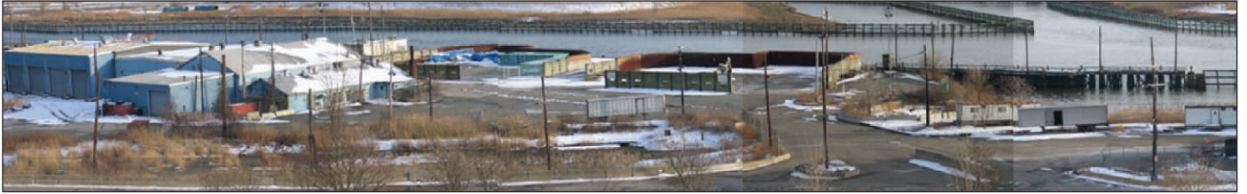
DSNY operations-related buildings on site 7
