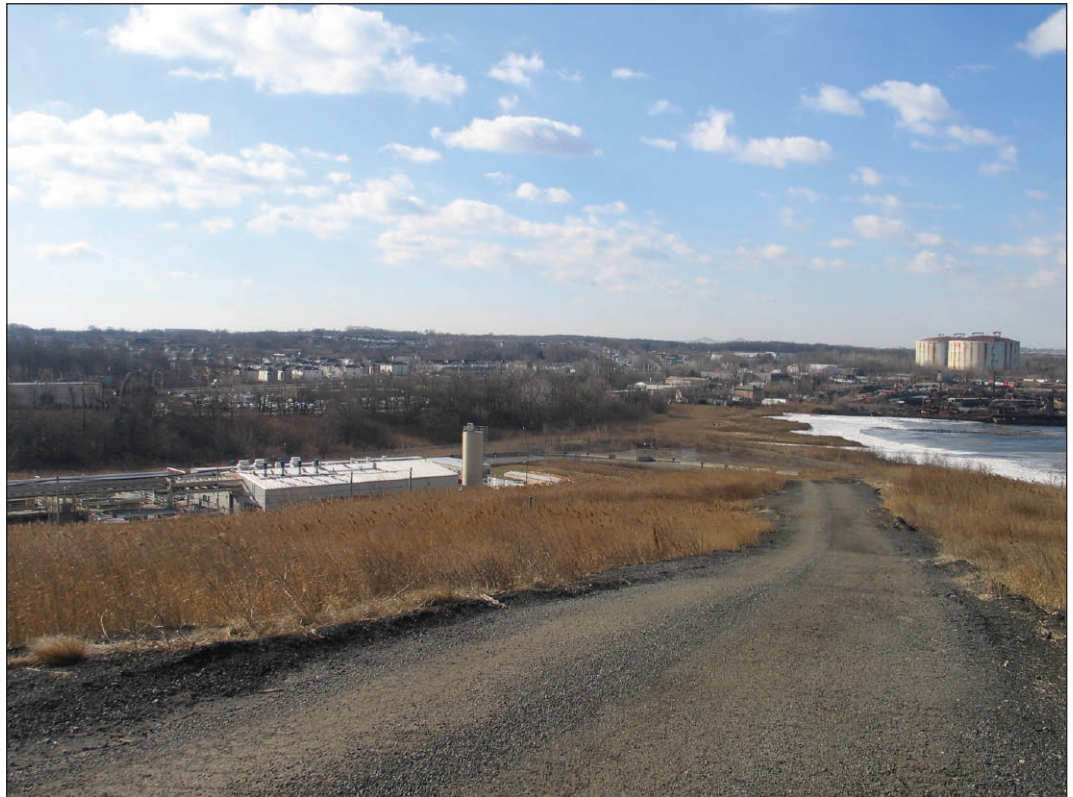
Unpaved truck route (view south from 1/9) 4
