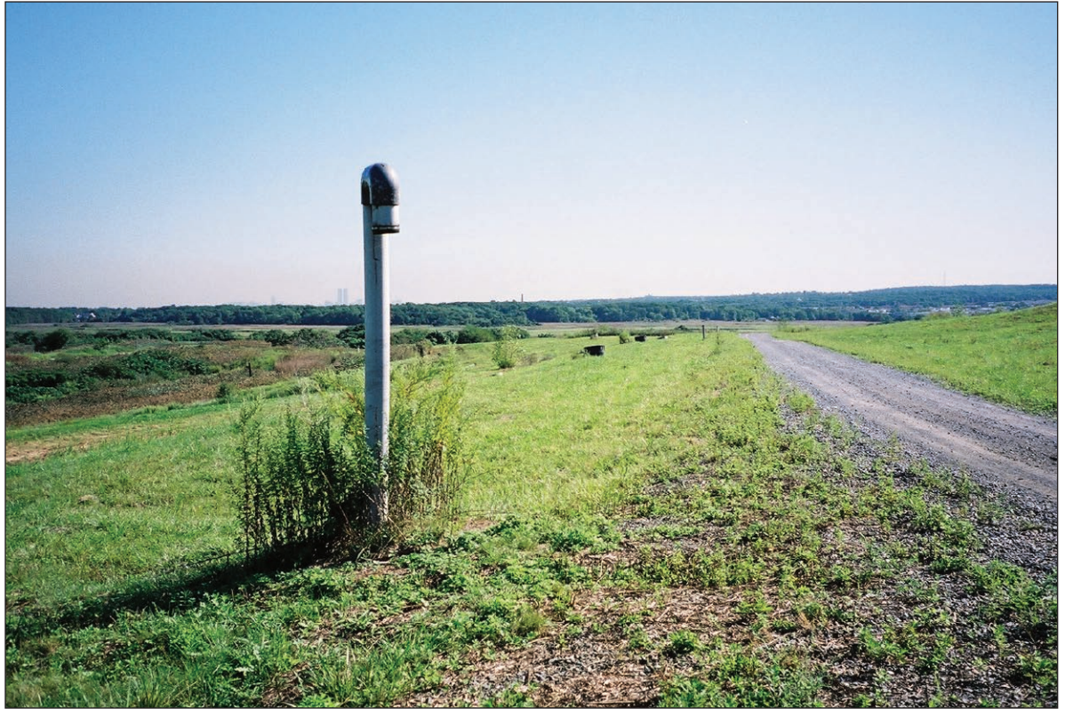
Above-ground infrastructure networks have a visual presence on site 12
