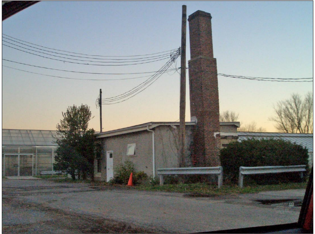
Another building, once used as a potting shed and heat generating facility, located on the former Mohlenhoff Farm, is now the NYCDPR native plant center. Greenhouses built prior to 1937 are visible on the left and right 5
