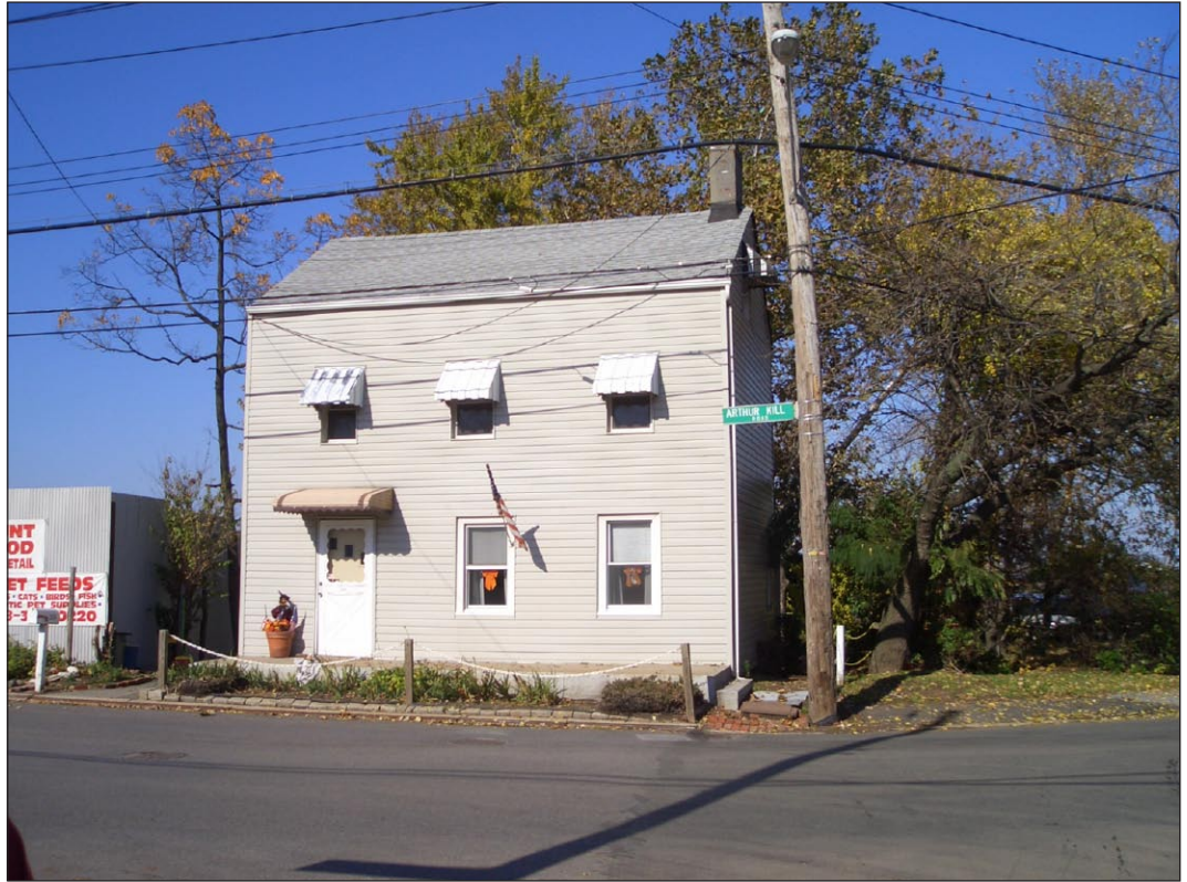
The former Winant House, 2341 Arthur Kill Road, located at the head of Rosville Avenue on the north side of Arthur Kill Road. The residence has been altered in recent decades with the introduction of modern siding and retrofitted windows; however, the early vernacular structure stood at what was once the central crossroads of the town of Rosville
