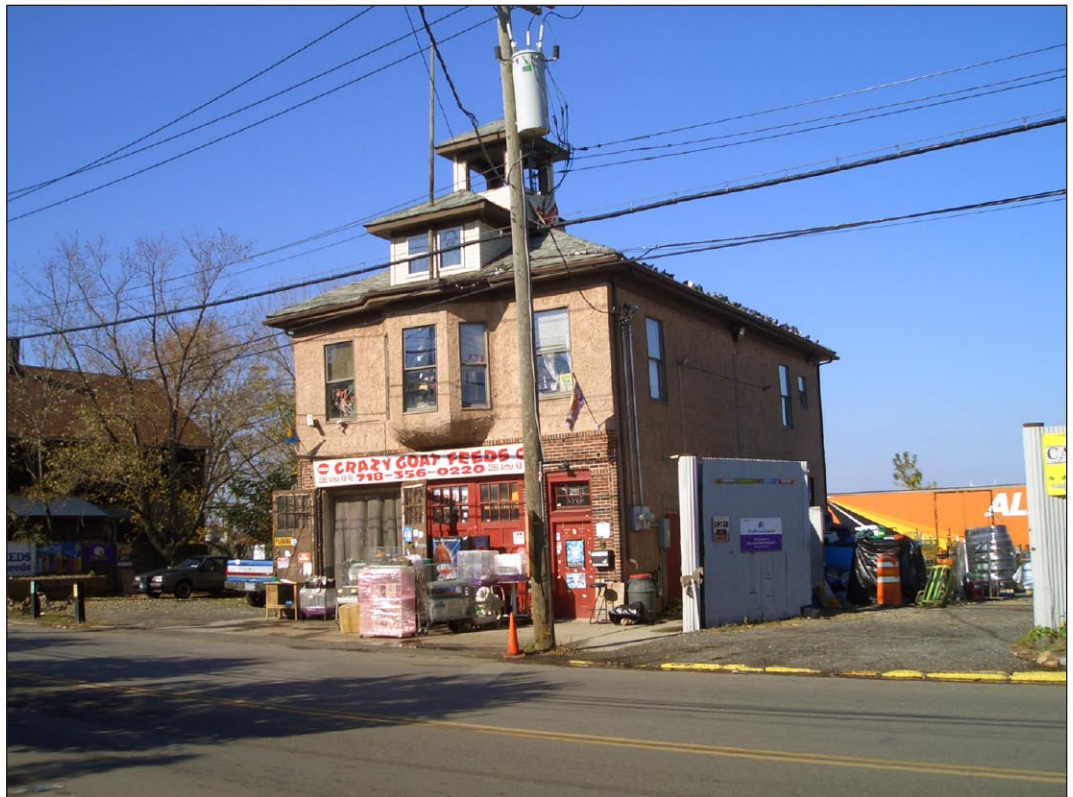
The former Rosville Hook and Ladder firehouse at 2355 Arthur Kill Road retains its large central doors and bell tower, but has been parged with stucco and received retrofitted windows. The structure is now a feed store
