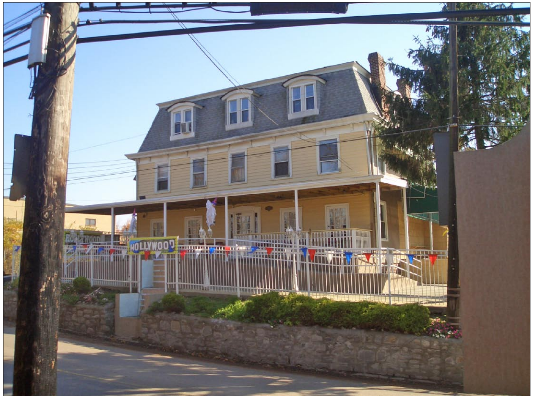
The Second Empire-style structure at 2285 Arthur Kill Road, built ca. 1860 on the south side of 10 Arthur Kill Road in Rossville. The former residence is now a nightclub
