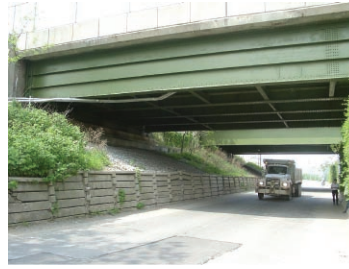
SOUTH UNDERPASS LOOKING WEST
