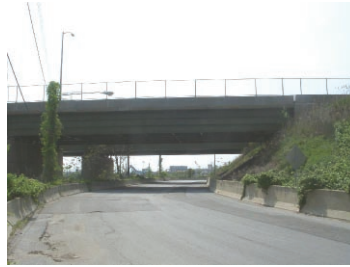
NORTH UNDERPASS LOOKING WEST
