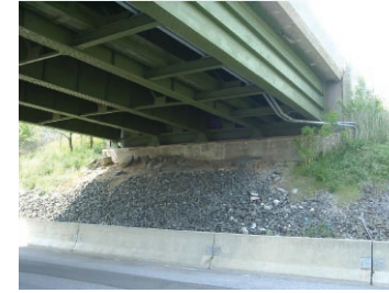
NORTH UNDERPASS LOOKING NORTH
