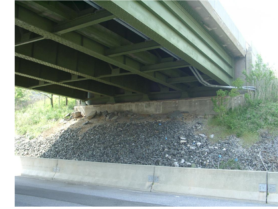
NORTH SIDE LOOKING EAST
