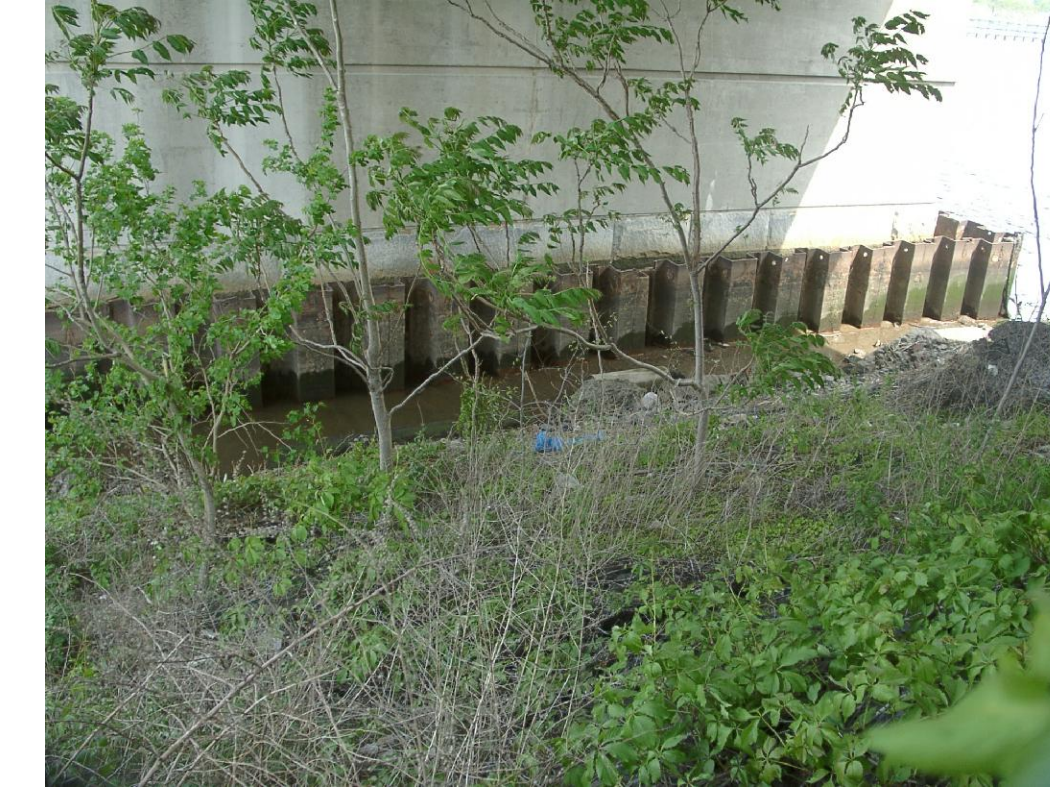
SOUTH SIDE LOOKING EAST
