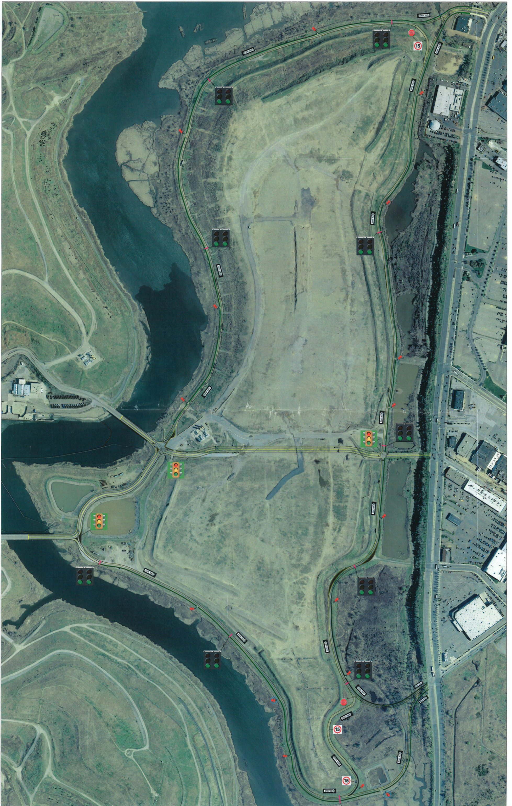
FRESH KILLS LANDFILL AERIAL VIEW WITH BOROUGH PRESIDENT'S DESIGN UTILIZING EXISTING HAUL ROADS ADJUSTED TO TRAVEL STANDARDS (SECTION 6/7)
