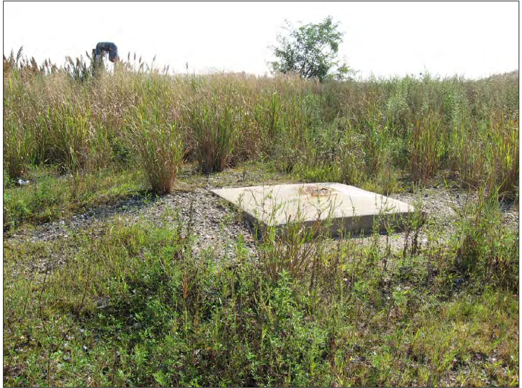
Examples of utilities at top of North Mound 9
