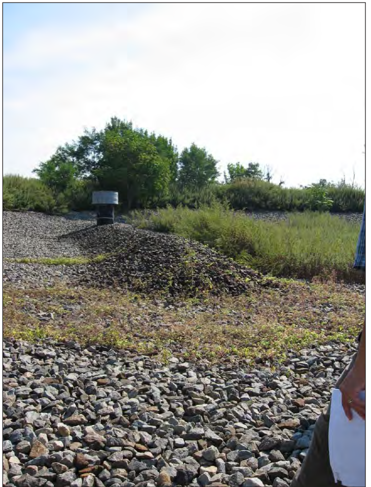
Stormwater drain within basin to north of North Mound, looking east 4
