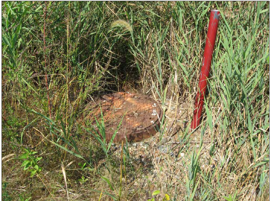
Typical manhole, at base of North Mound 10
