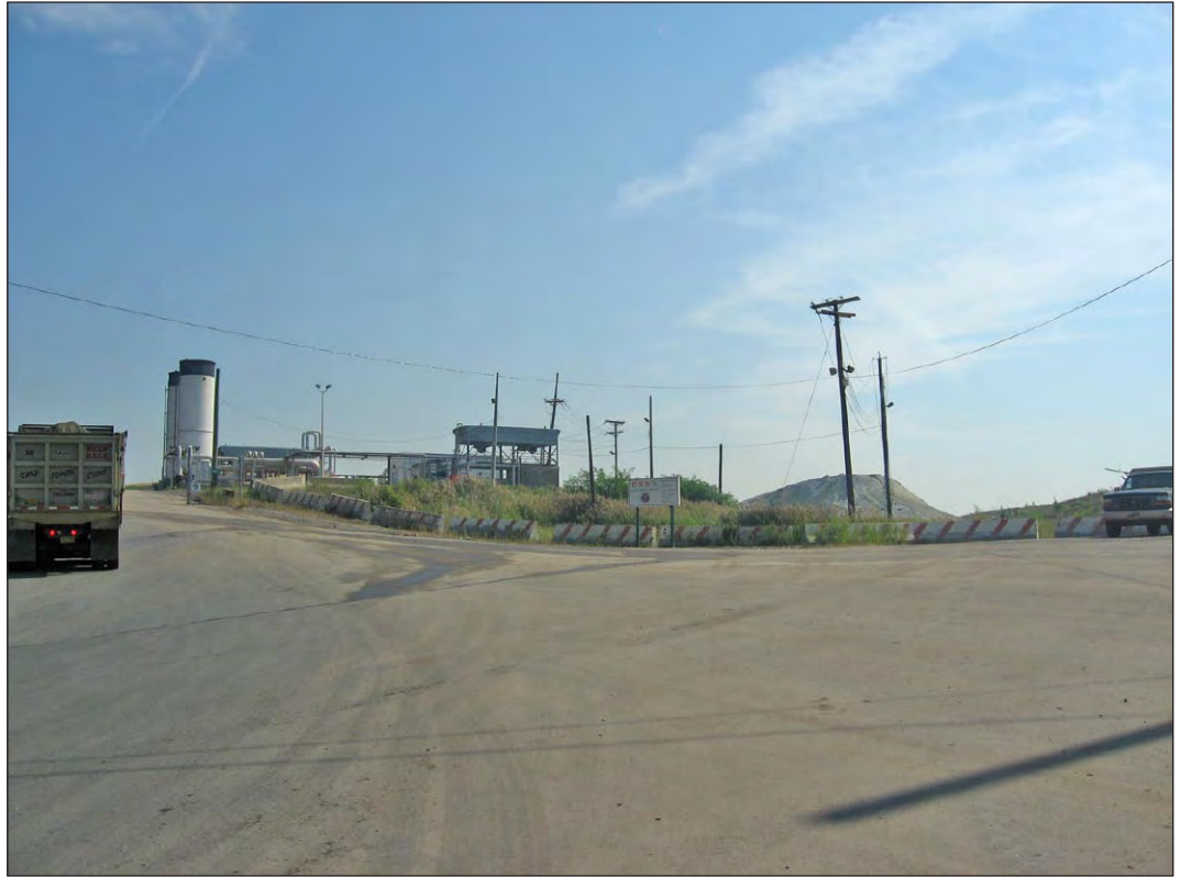
Flare Station on East Mound, looking northeast 1
