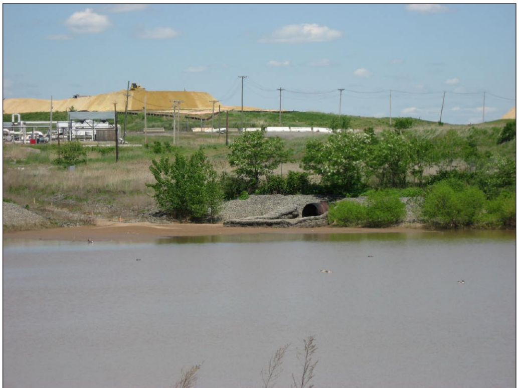
Large stormwater management basin at the Convergence of Main Creek and Richmond Creek 8
