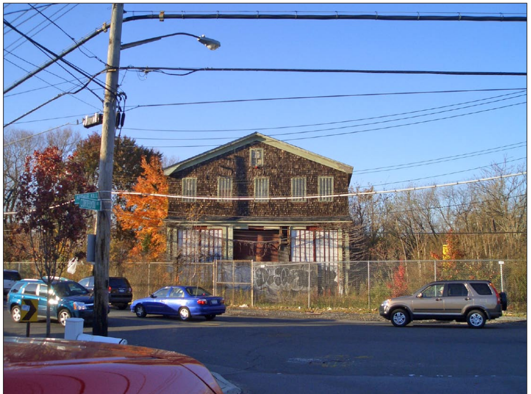
Located at 721 Arthur Kill Road, this former trolley barn originally served the Tottenville and Richmond Trolley. This building was determined S/NR - eligible as part of this project 6
