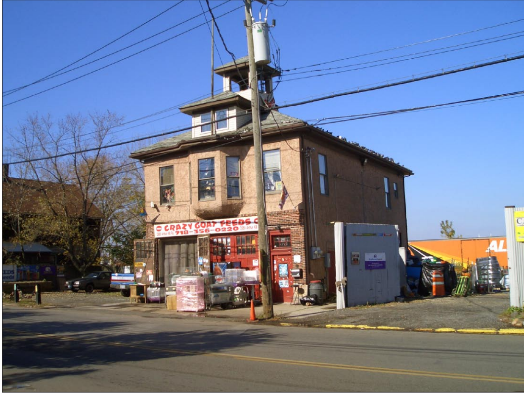
The former Rossville Hook and Ladder firehouse at 2355 Arthur Kill Road retains its large central doors and bell tower, but has been parged with stucco and received retrofitted windows. The structure is now a feed store. It was determined S/NR - eligible as part of this project 8
