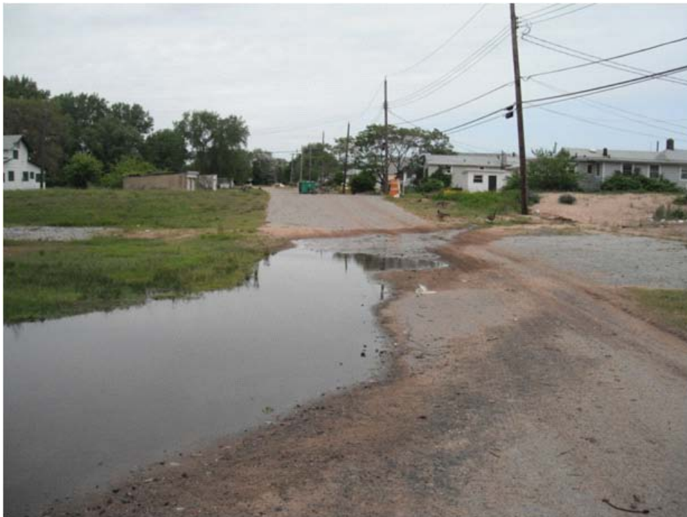
Photo 10 – Water flowing from a broken distribution line observed on June 5 and 6, 2011.
