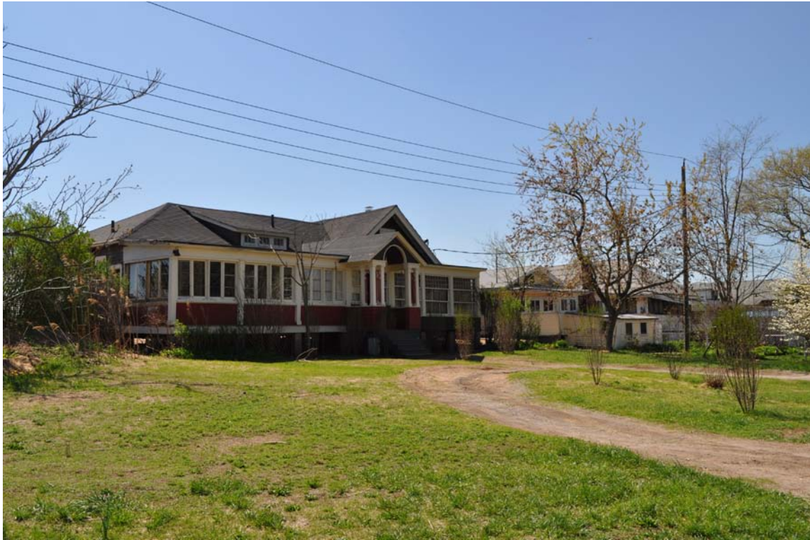
Photo 3: Looking southeast toward Building 4 which may be reused as the Public Concessions Building under the Proposed Action.
