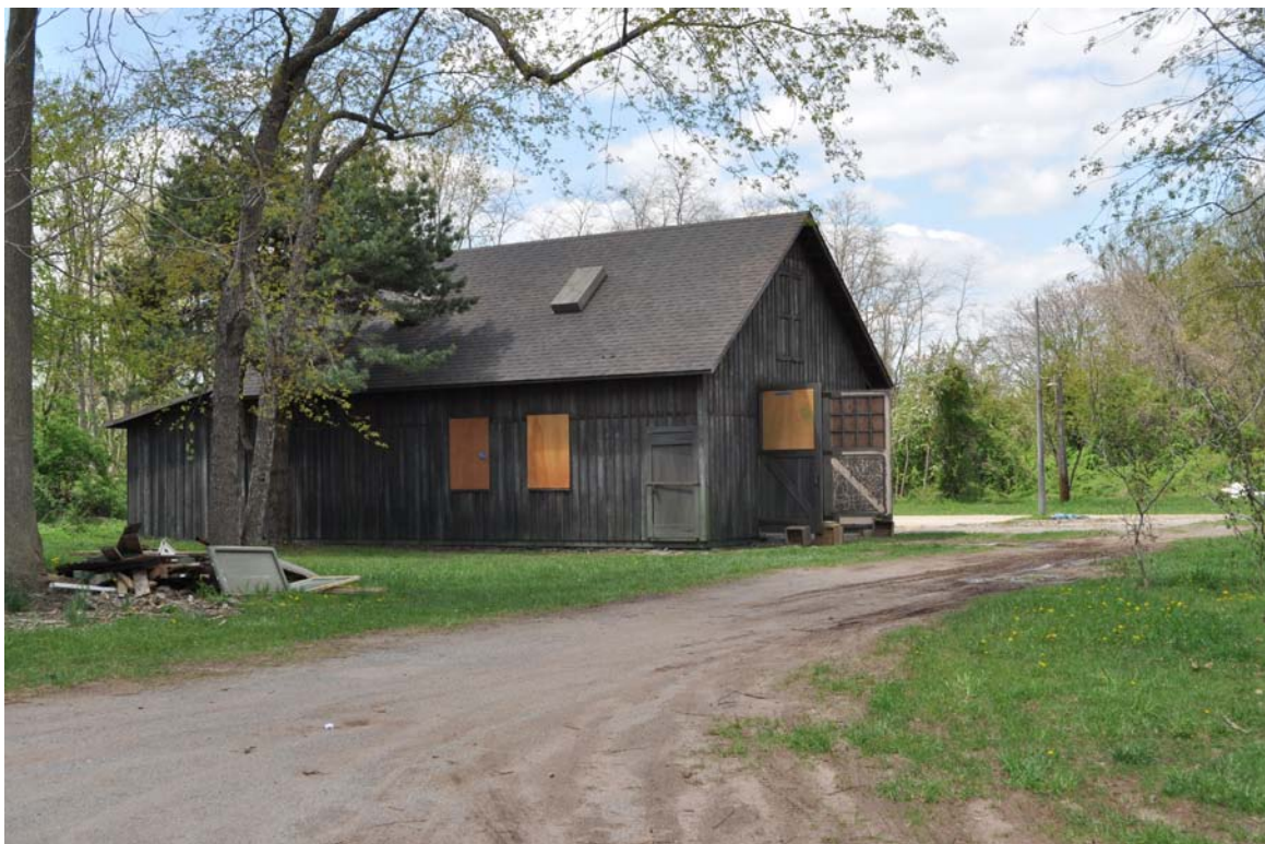
Photo 8: Looking north toward the Barn which may be reused as the Storage Building under the Proposed Action.
