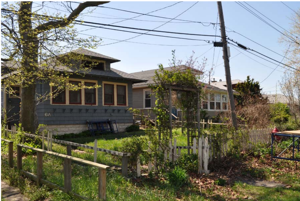
Photo 4: Looking east toward Building 6A (left) and Building 7 (right). Building 7 may be reused as the Lifeguard Station under the Proposed Action.
