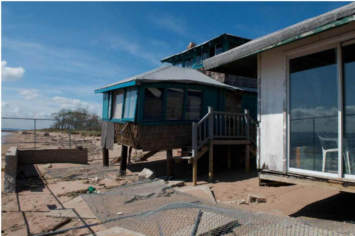
Photo 2: View of damaged bungalows looking south along Cedar Grove Beach.
