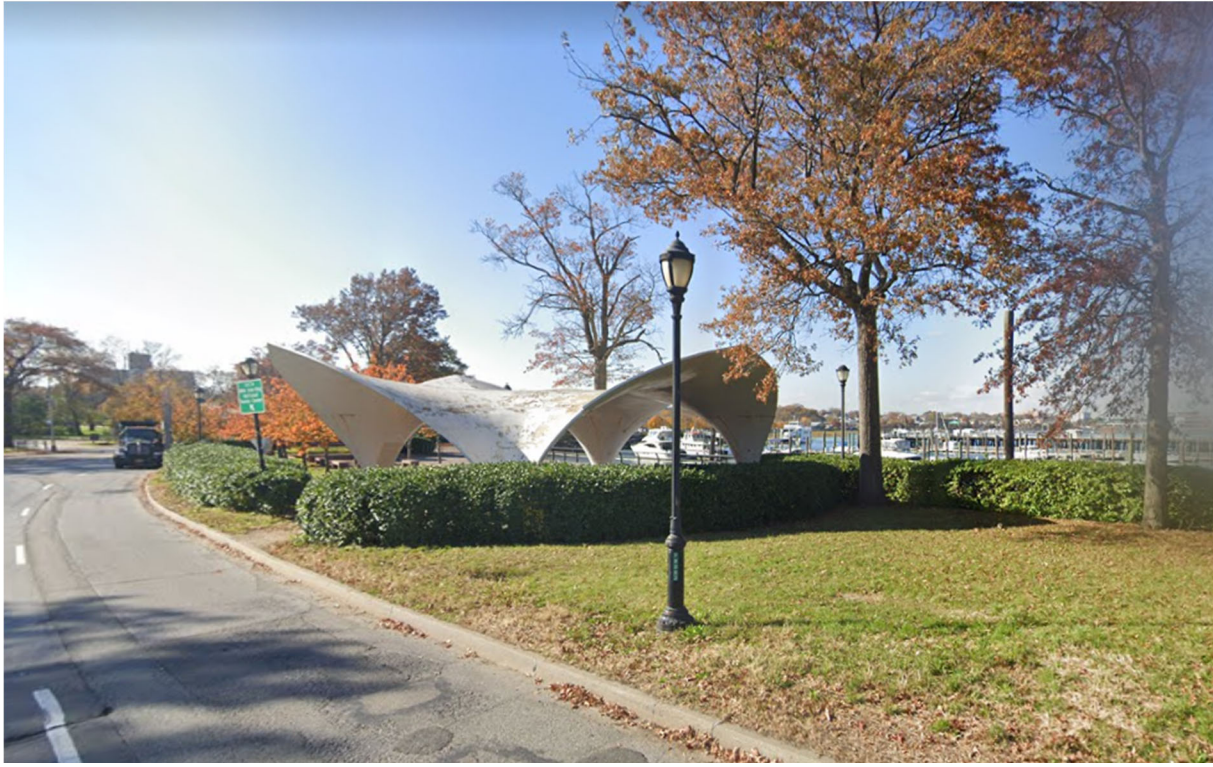
Fig. 3. Image of Candela Structures adjacent to Pier 1. Image via Google Street view.
