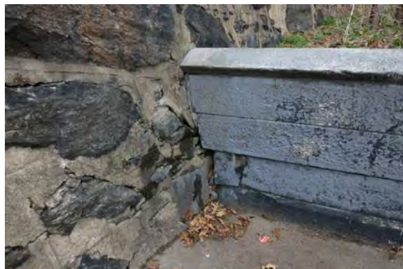
12 VOIDS & MATERIAL LOSS
