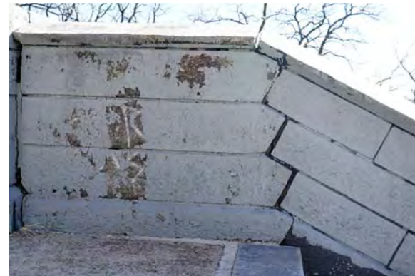
9 STEP CRACK
