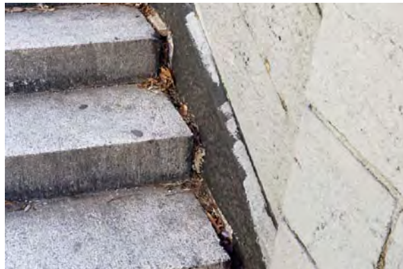
3 MISSING MORTAR
