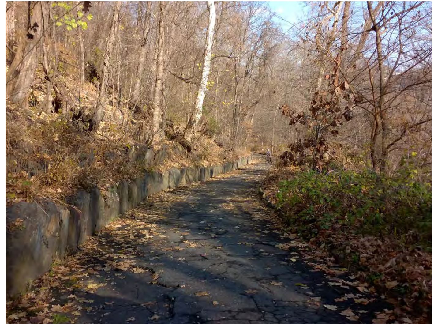
10 - A series of stone terraces occurs along a narrower portion of the path (12' wide) in which trees have volunteered over time. Poor pavement condition is typical along this northern section.
