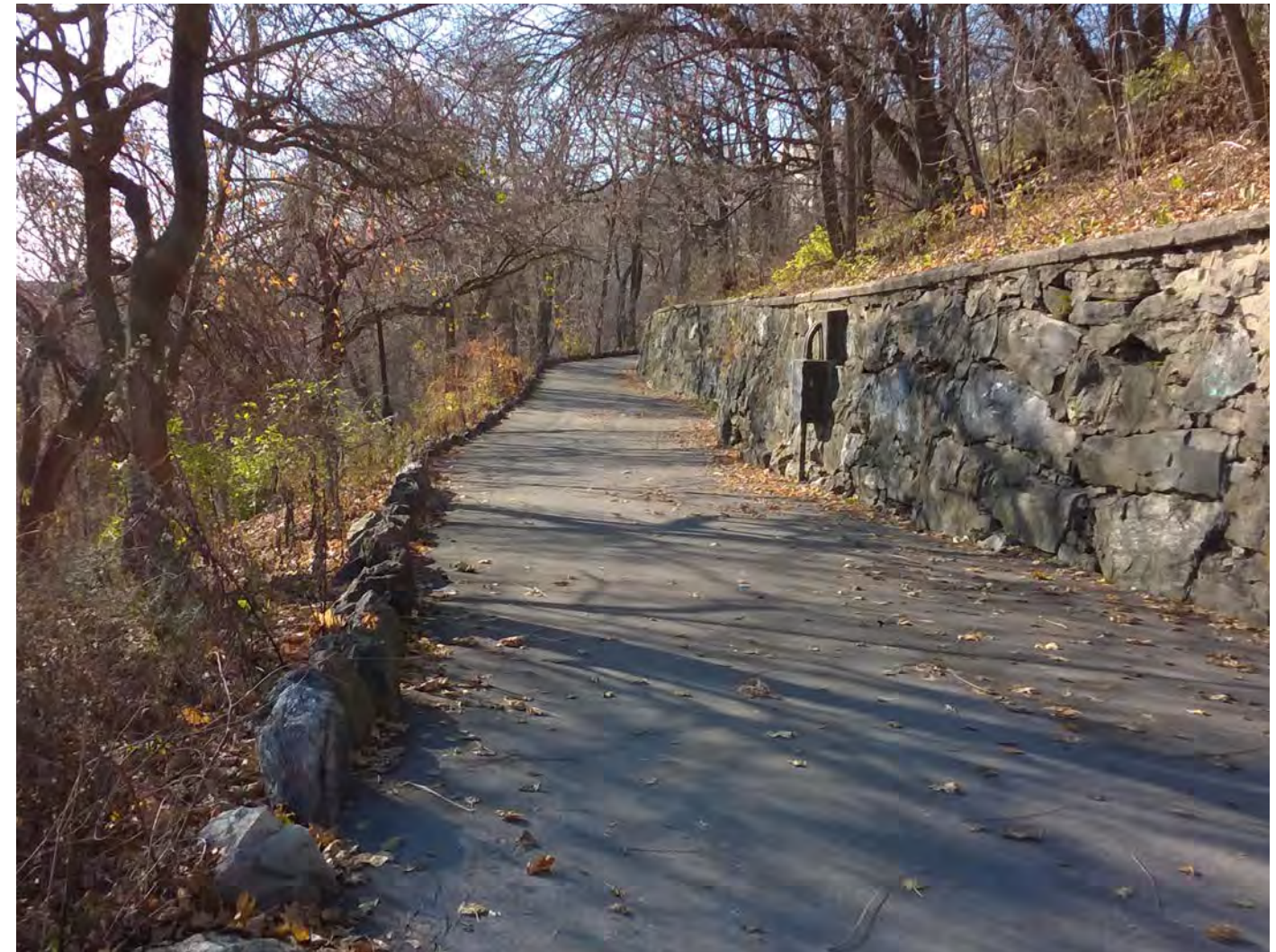
6 - Typical pathway alignment, grade and adjacencies of rubble stone walls and curbs.
