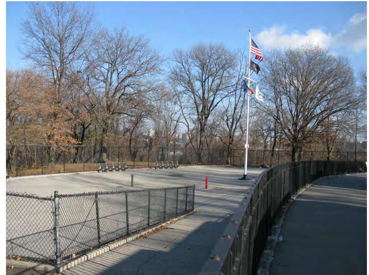
7 - A portion of Fort George Playground illustrating the expansive spray shower area.
