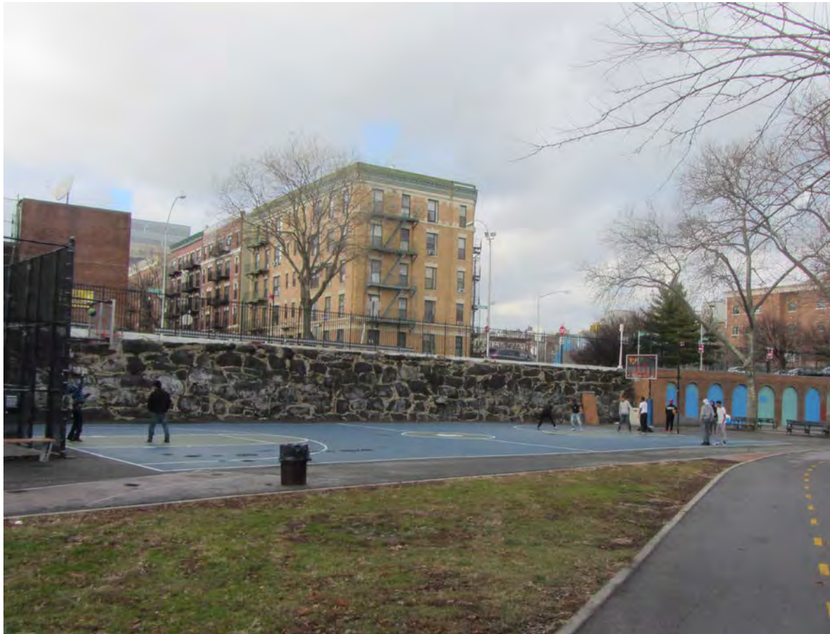
3 - Sunken Playground consists of handball and basketball courts and sitting areas well below the adjacent sidewalk grade.
