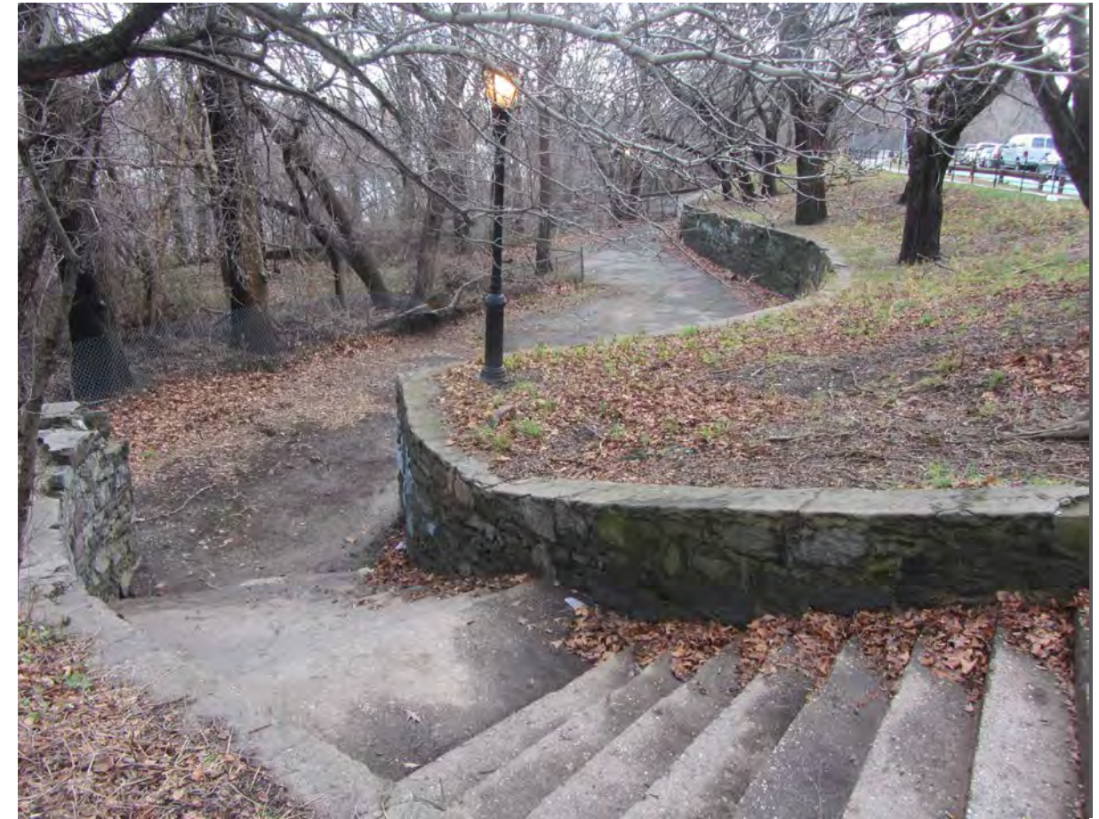
4 - Steps down into a depressed area along Edgecombe Avenue, originally designed as horseshoe pitches.
