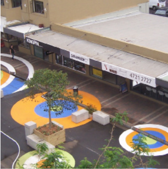
The space is now complete and useable but evolving as new information comes on board. Vehicle access for deliveries and maintenance have been responded to and elements can be modified to meet new demands on the space.
