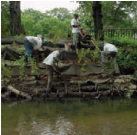
Above: Members of the Bronx River Alliance and volunteers are transforming the Bronx River. Here, crew members stabilize the riverbank using terracing and planting.
