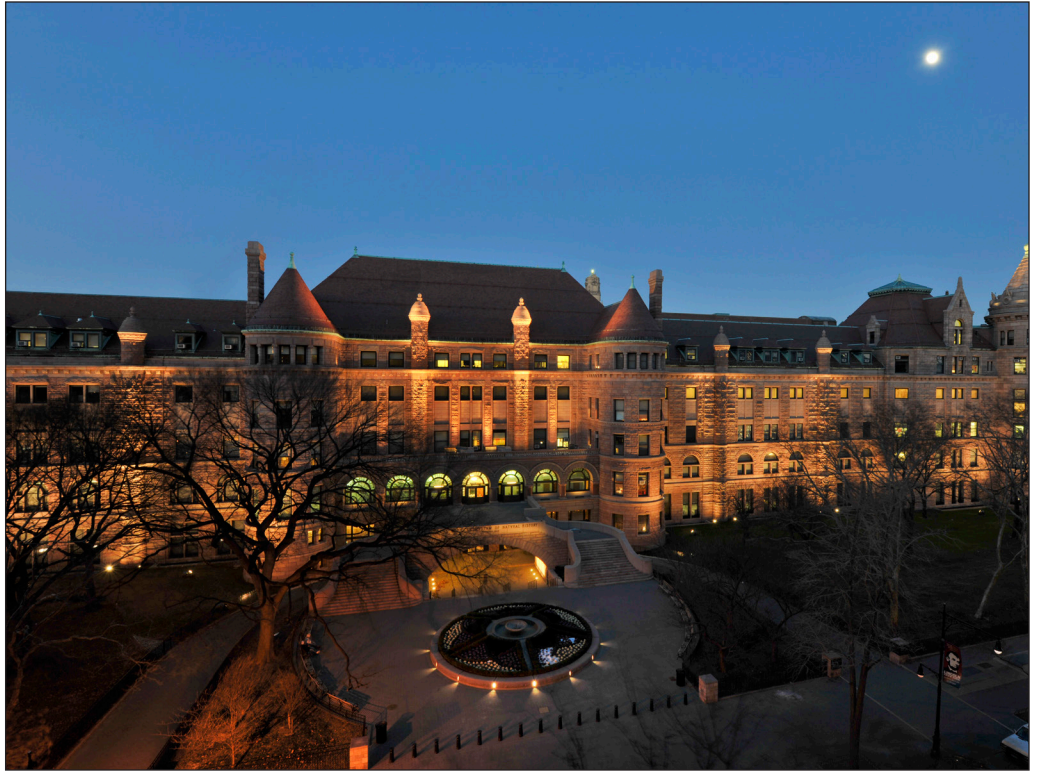
Evening View of West 77th Street Entrance
