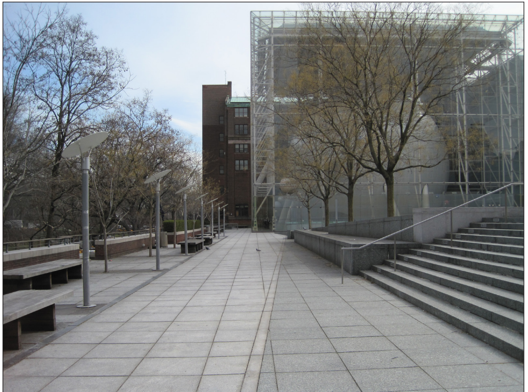
AMNH. View east on Ross Terrace 8
