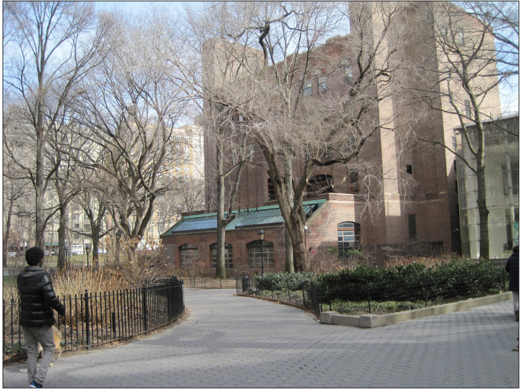
AMNH. Former power house. View northeast 3
