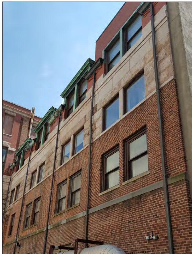
View of the north façade of Building 15 10
