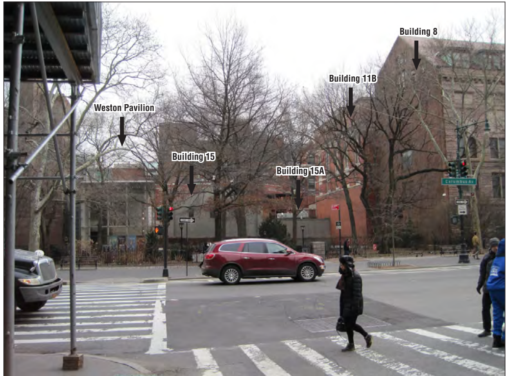
View east of the Museum from Columbus Avenue including the Weston Pavilion, Building 15 (the former power house), Building 15A, the north façade of Building 8, and the north façade of Building 11B
