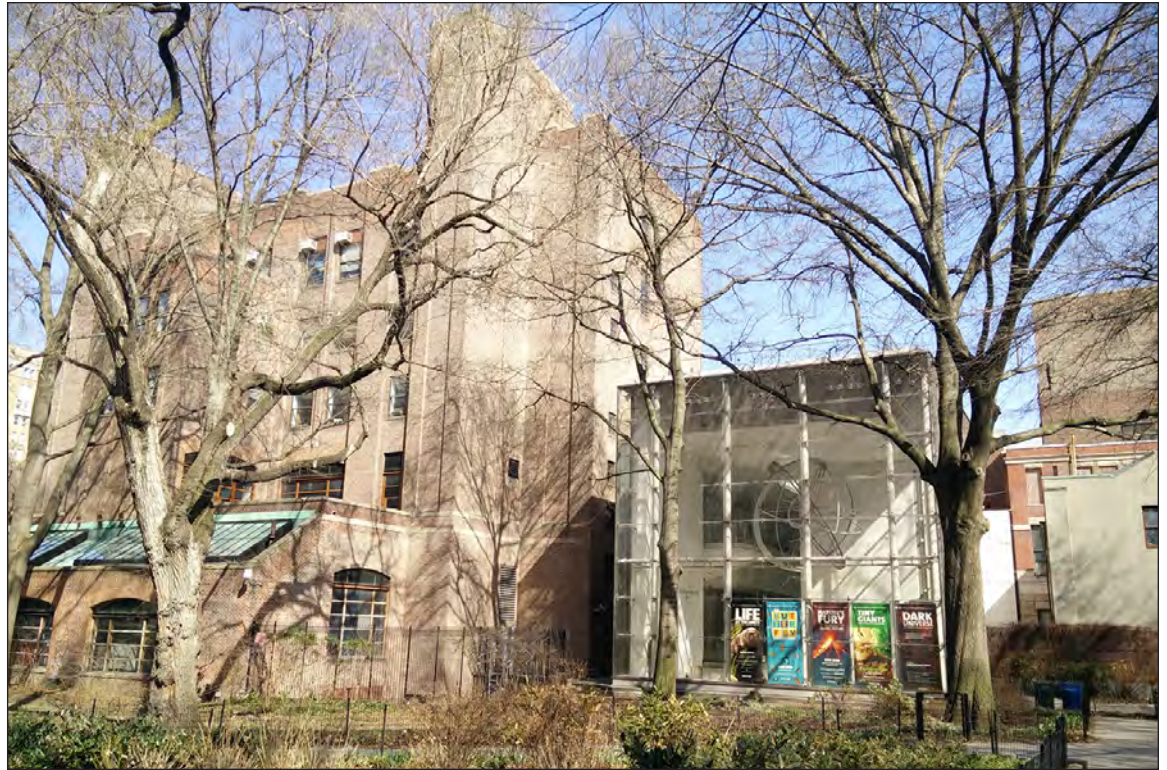
View of Existing Building 17 and Weston Pavilion 5
